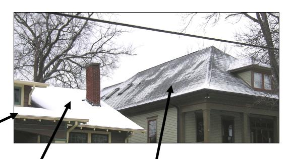
No melted snow here...they have attic insulation.
