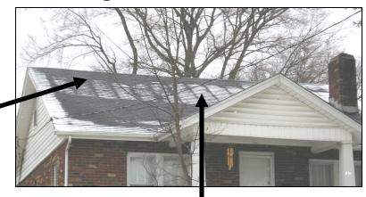
These lines are the 2x roof rafters, which are transferring the heat to the roof.
